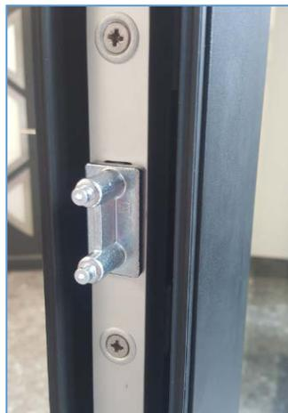
3. Slide the door shut, firmly but not too hard. This will mark two points on the outer frame jamb. Fix the locking keep into these points after drilling a 4mm hole where marked and using the screws provided.
